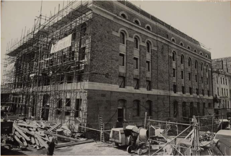
Figure 5. Bush House renovation (exterior), November 1974 (Bristol Archives re. no: 43371/Adm/3/4/2/4).
